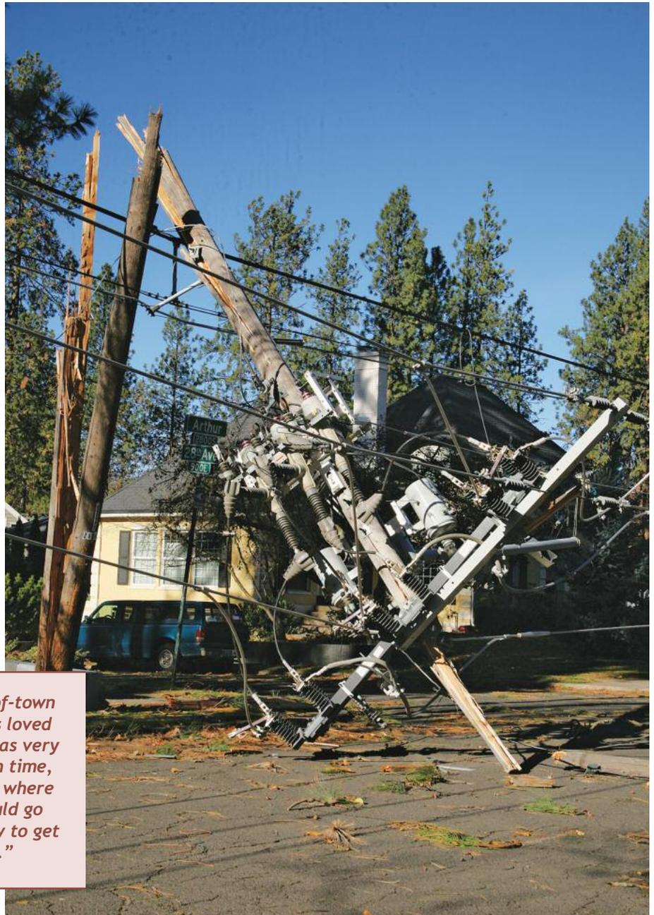
*Broken poles and sagging lines, often caused by wind-damaged trees, made it difficult to drive in parts of Spokane until Asplundh and Avista could clear roadways.*
