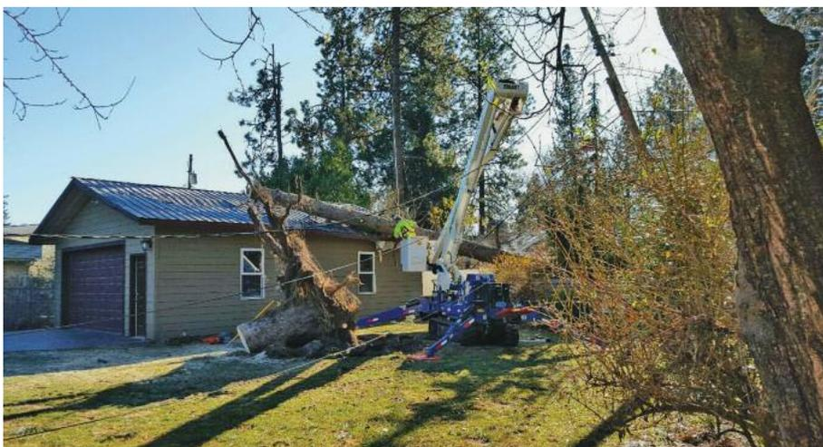
*After the November 17, 2015 storm, Asplundh Foreperson Matt Nelson maneuvers a backyard aerial lift into position to carefully remove a pine that pulled down Avista's primary and secondary power lines.*
